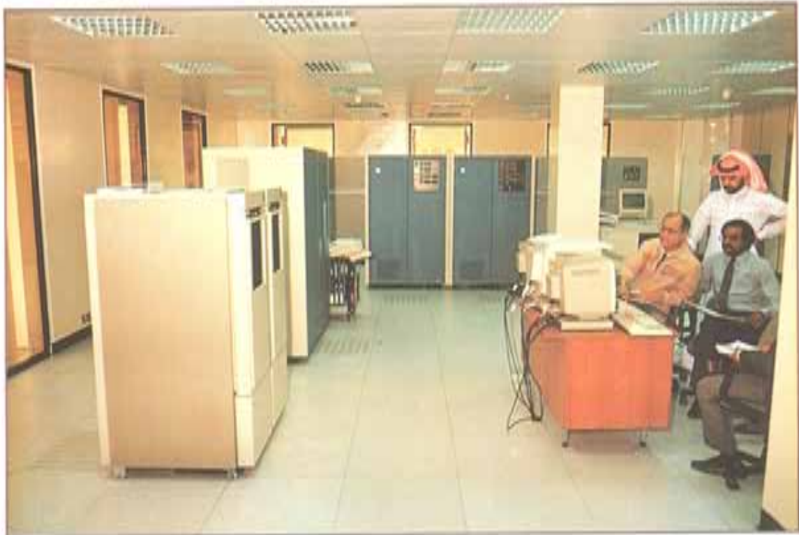
Computer Operation Room in Qatar National Bank
