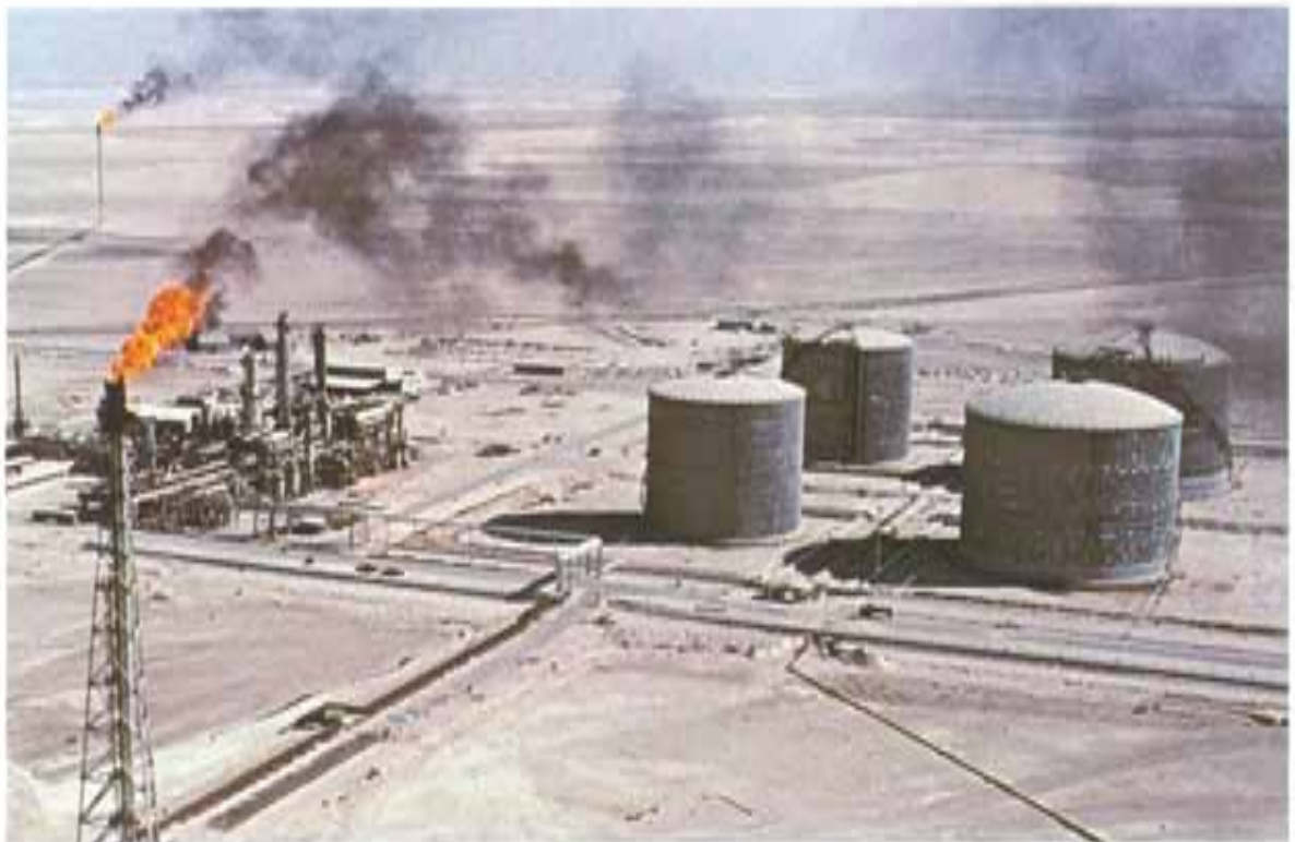
National Gas Liquefaction Plant
